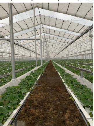
On a hot day the roof is opened 50 cm in each bay to allow venting, while blocking UV (Photo credit: Jim Ripepi)
